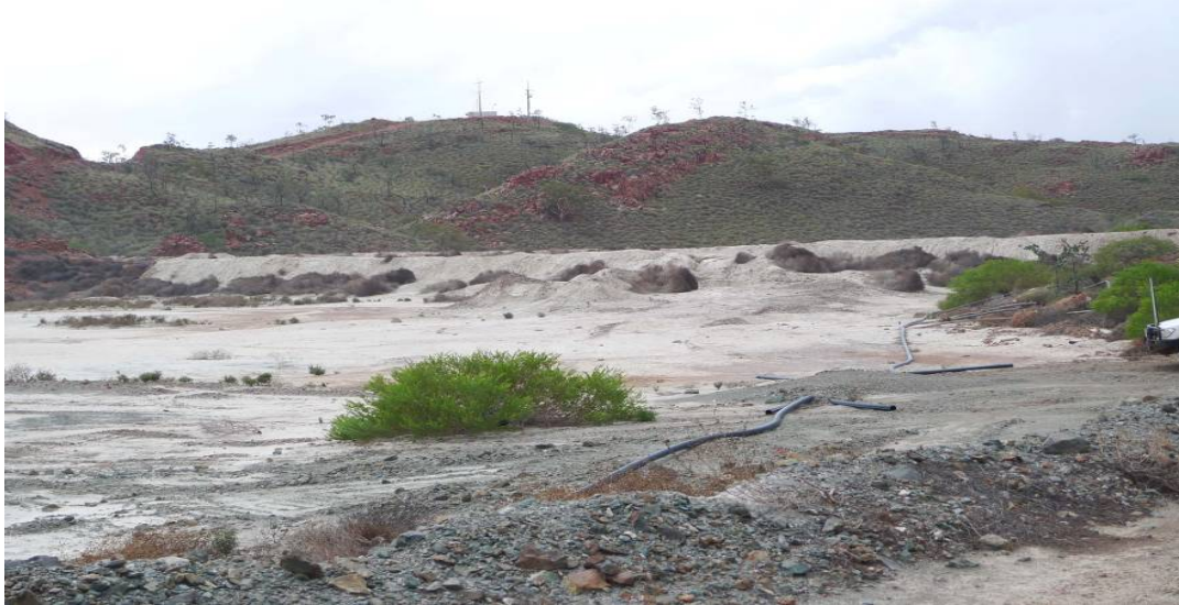
Figure 1: Bamboo Creek Tailings Dam
