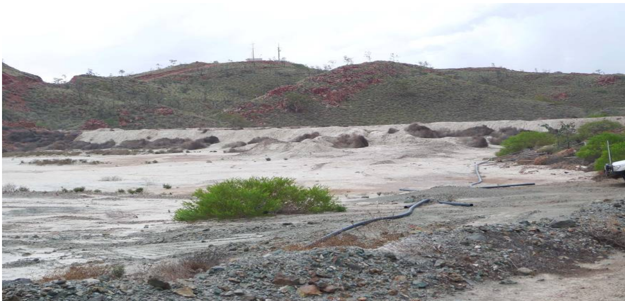
Figure 2: Bamboo Creek Tailings Dam
