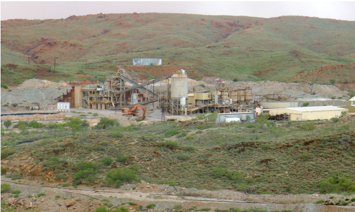
Figure 1: Bamboo Creek Processing Plant
