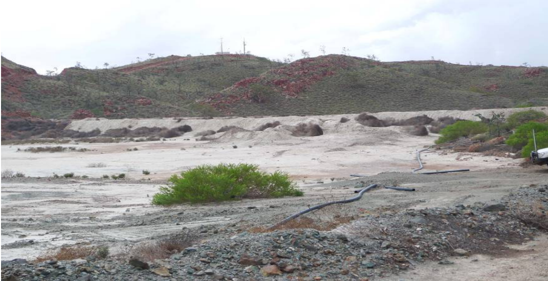
Figure 1: Bamboo Creek Tailings Dam
