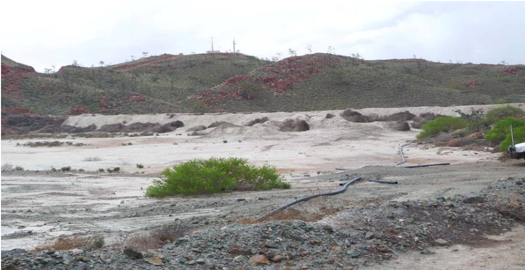
Figure 1: Bamboo Creek Tailings Dam
