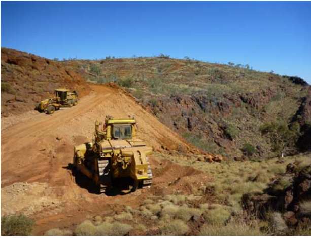
Figure 2: Mt Webber northern access ramp construction.
